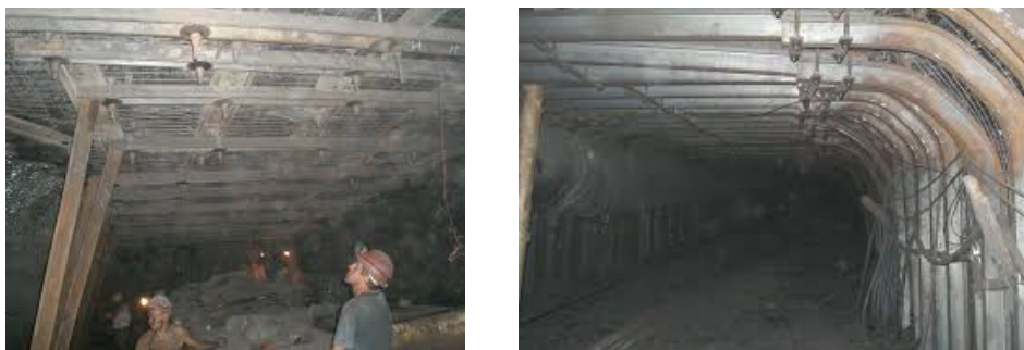
Fig. 1. View of bearing structures of the building.
