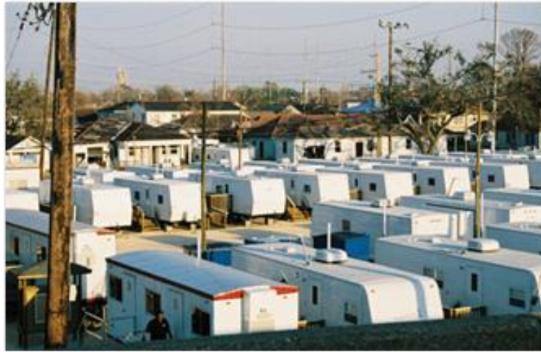
Figure 5. Trailer Park, (USA, 1960s)
