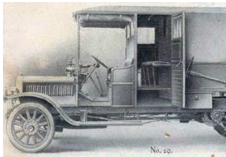
Figure 3. Sleeping compartment in the cab of a Gaggenau truck (1910).
