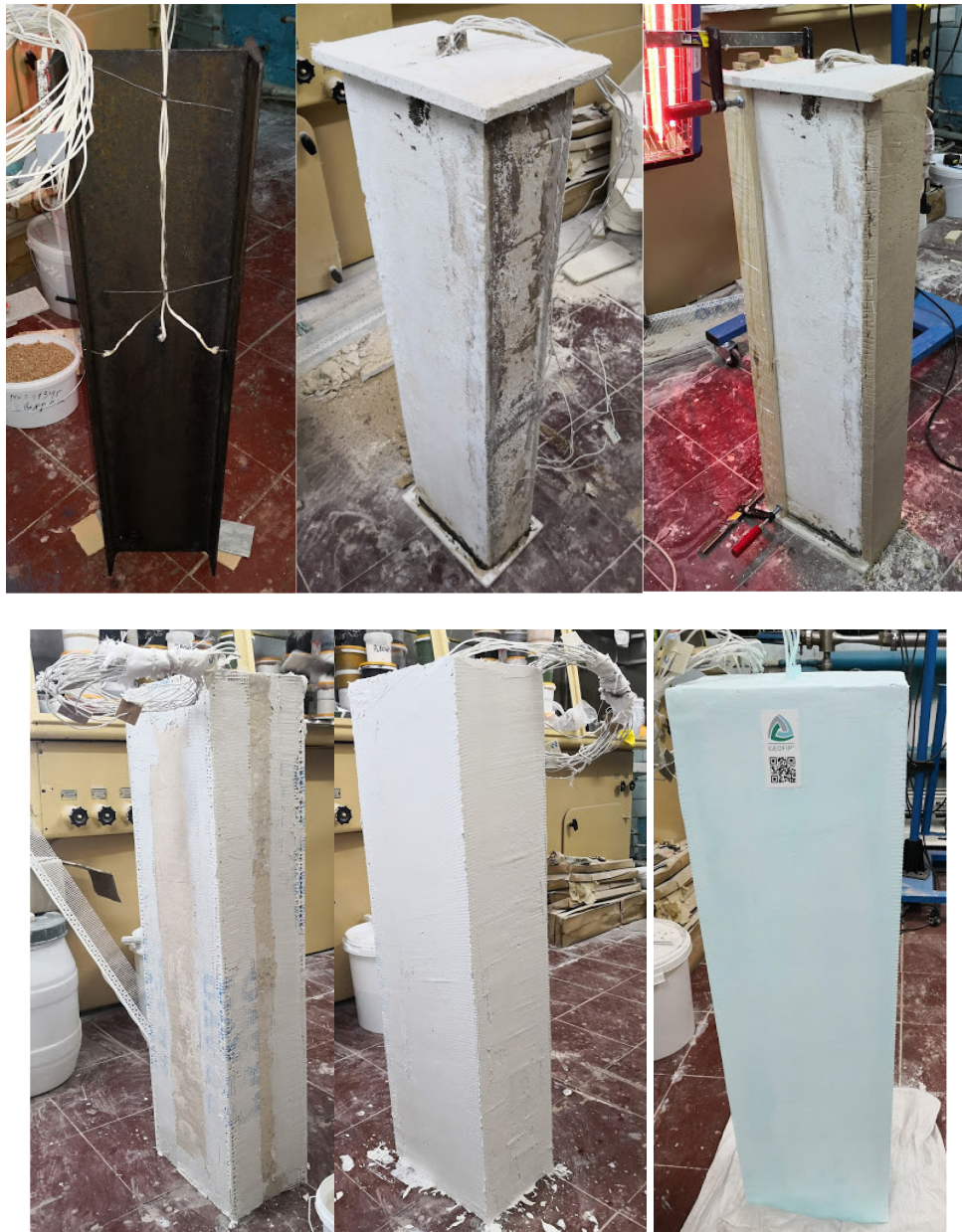
Fig. 2. Snapshots of the work stages during the preparation of an I-beam for fire test
