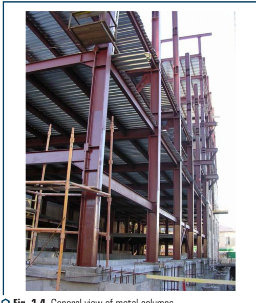
○ Fig. 1.4 General view of metal columns
