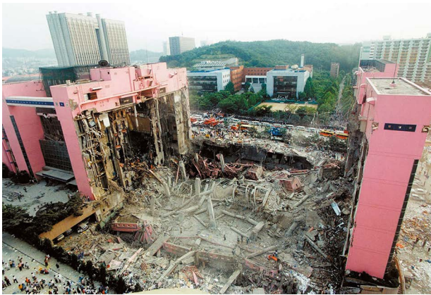
○ Fig. 1.9 Collapse of a 5-storey supermarket in Seoul, 1995
