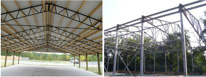
○ Fig. 1.3 General view of the steel truss
