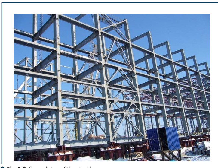
◉ Fig. 1.2 General view of the steel beam
