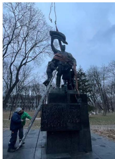
Figure 3. The dismantling of the monument to the armed January uprising of the Bolsheviks in 1918.
