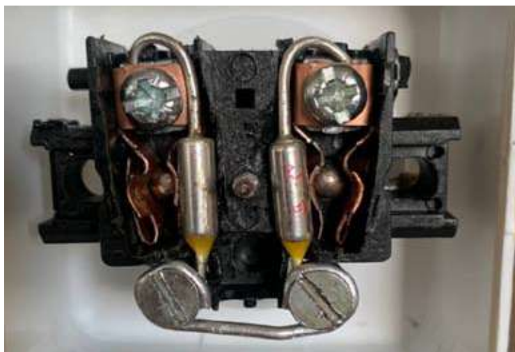
Fig. 2 : Socket with thermal fuse
