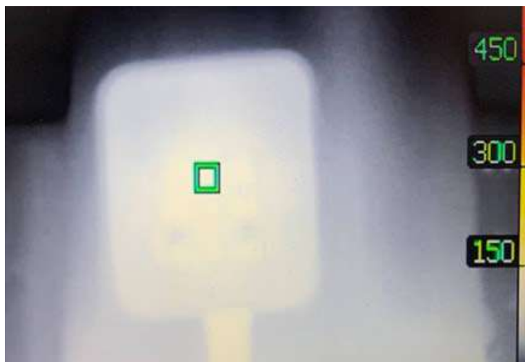
Fig. 4 : An example of temperature distribution (°C) in an electrical load element under the conditions of an oxidized plug and a normal socket
