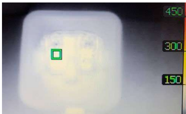
Fig. 6 : Example of temperature distribution (°C) of an electrical load element under conditions of unsatisfactory contact and an oxidized plug.
