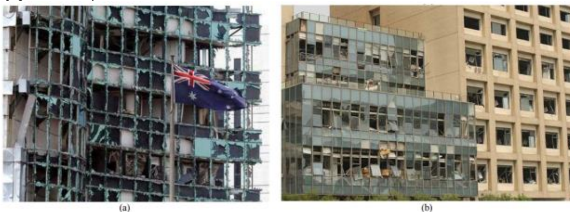
Fig. 1. Shattered glass windows. Examples referred to (a) the Australian Embassy in Jakarta, 2004 (photo by AP) and (b) Tianjin (China) explosive event, 2015, with evidence of framing systems ejection (photo by Wang Zhuangfei/China Daily)
