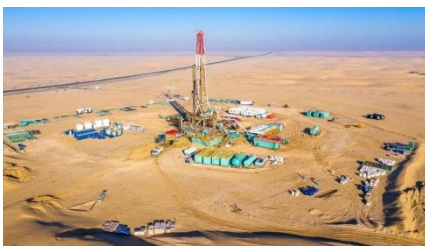
Fig. 2. An aerial view of the Jebel Ali gas field.
