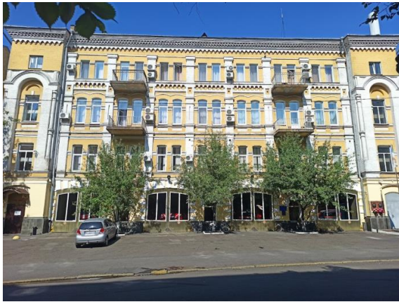
Fig.4. Solomyansk District Office of the Main Office of the State Emergency Service of Ukraine in Kyiv. The former depot building of the Lybid Fire Department, Kyiv [9]
