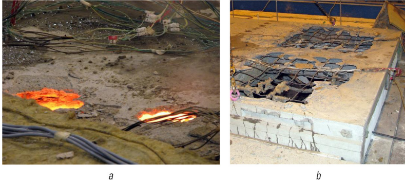
Fig. 3.14 The nature of the destruction of the panel of the ribbed reinforced concrete slab during its fire tests: a – during the fire tests; b – after the fire tests Source: [16]
