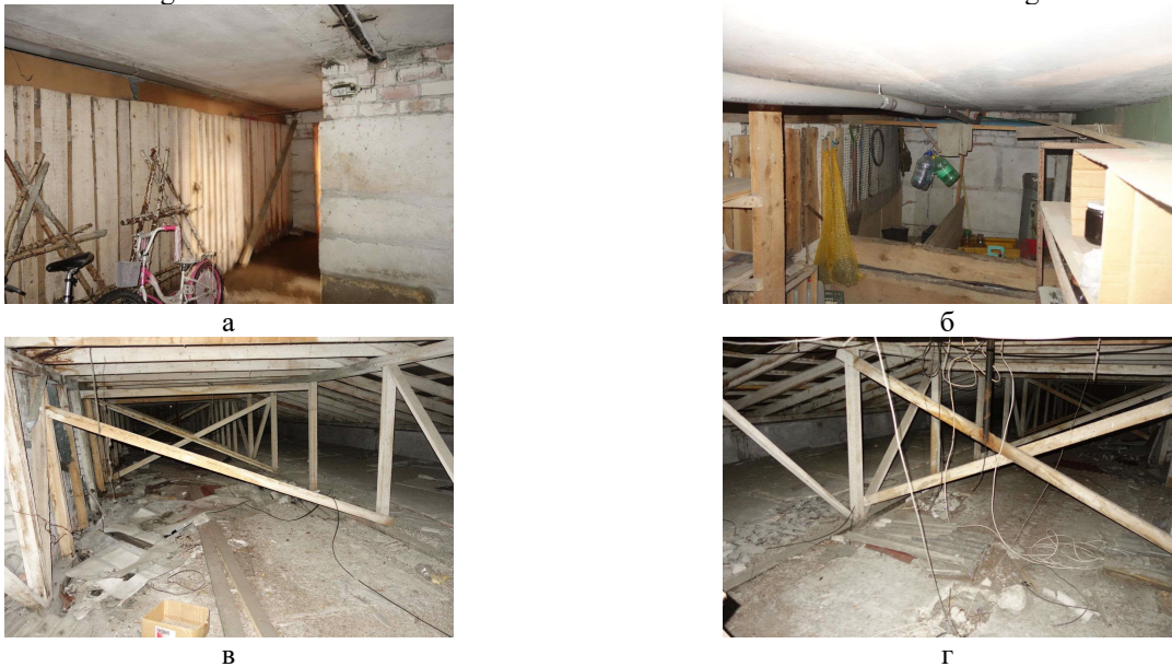
Figure 3 – Basement and attic of the hotel building
