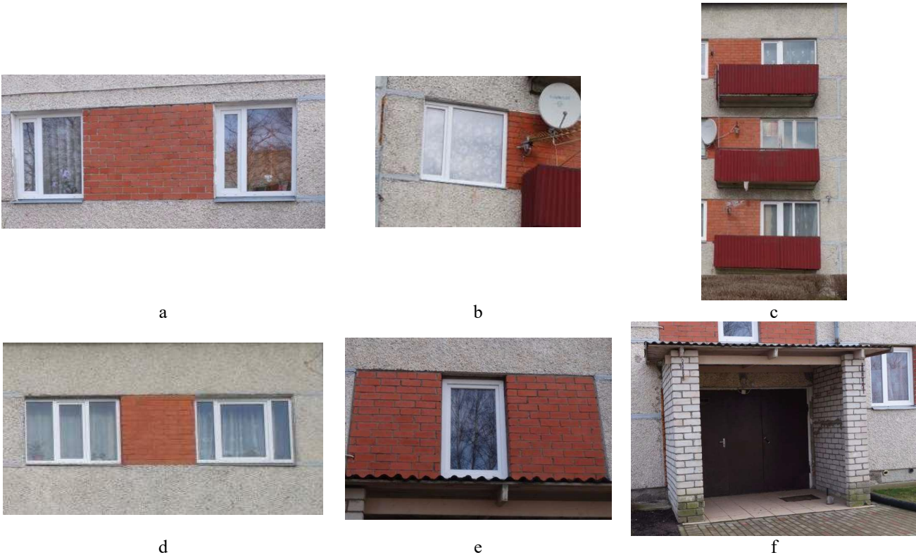
Figure 4 – Windows and entrance doors of the hotel building
