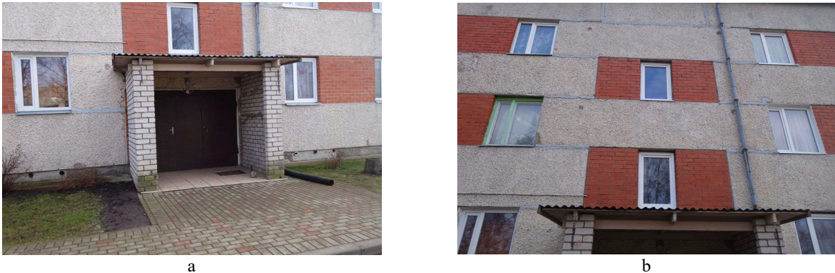
Figure 2 – Entrance doors and windows of the stairwells of the hotel building
