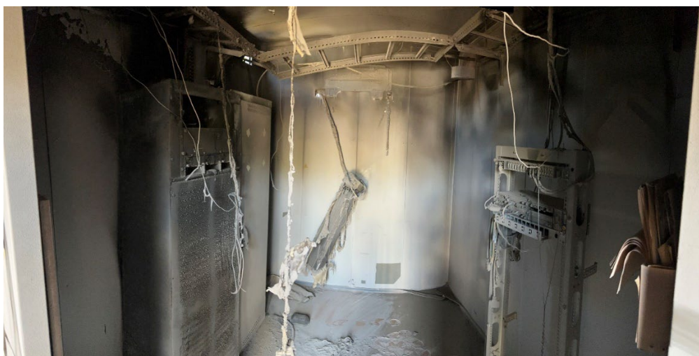
Fig. 13. Condition of the premises of the mobile communications base station caused by ignition of the 12V 100 A#2 batteries of the PSS SHZh power supply cabinet.
