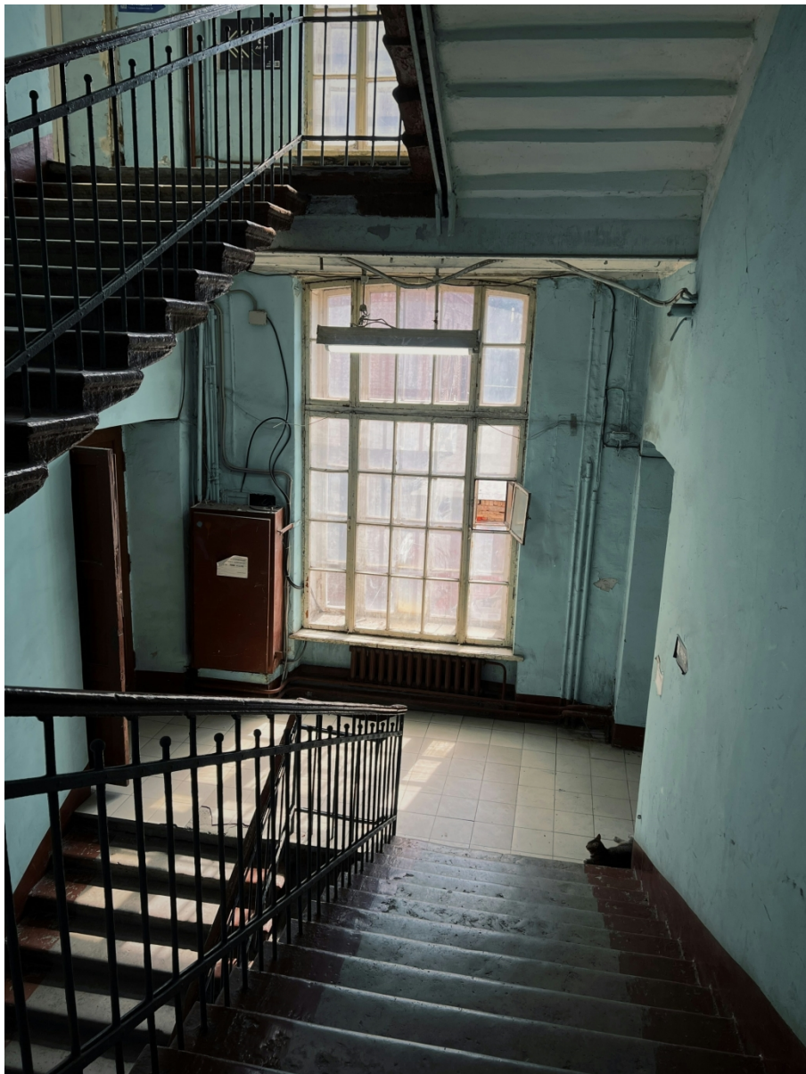
4.a. stairs with natural lighting
