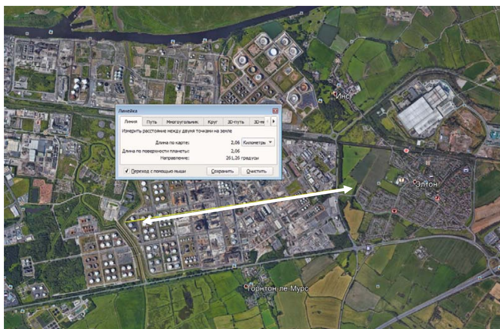
Fig. 1. Oil refinery photo
