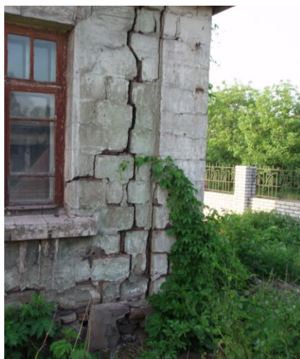
Fig. 2 – General view of existent building, located on investigated territories with the clearly expressed superficial cracks
