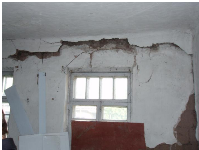
Fig. 2 – General view of existent building, located on investigated territories with the clearly expressed superficial cracks
